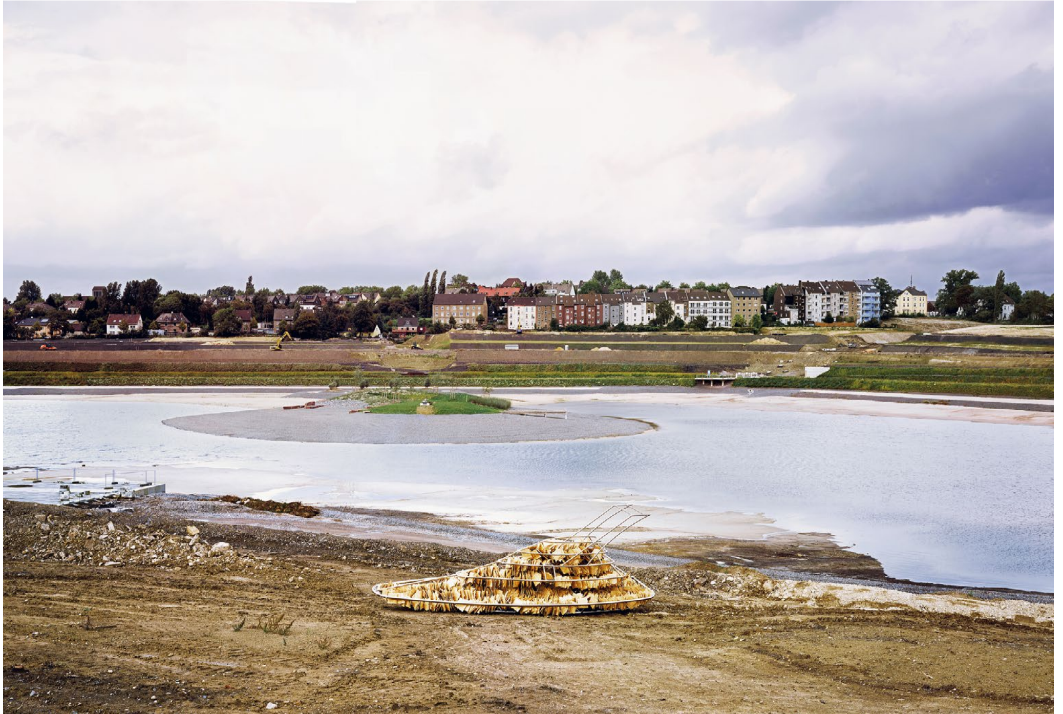
Site Photography - Temporary Harbour at LAKE PHOENIX 2010
